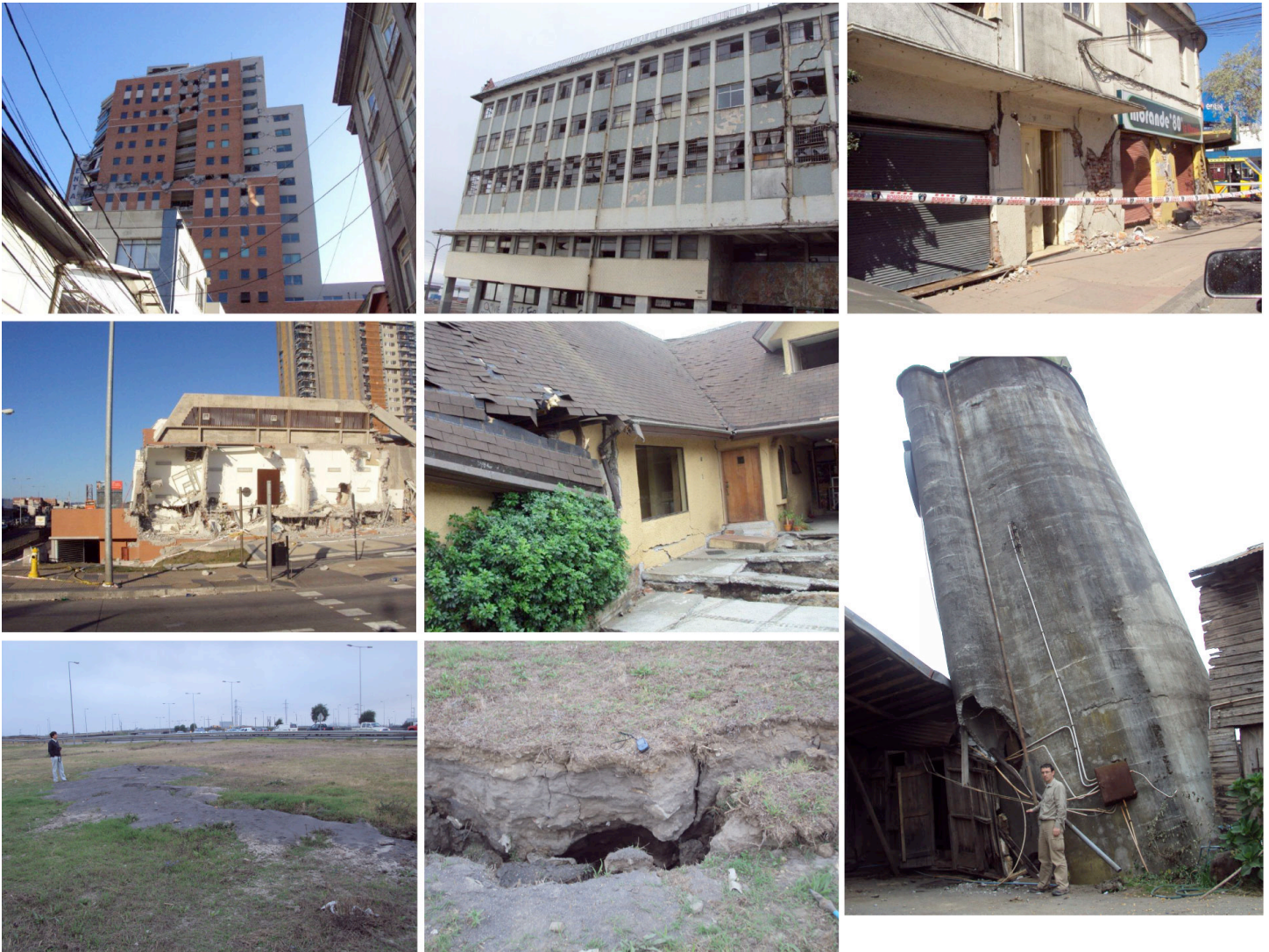
Fig. 5. Damage observed at the city of Concepción after the Maule 2010 large earthquake in: buildings, house due to lateral spreading, and evidence of liquefaction.
